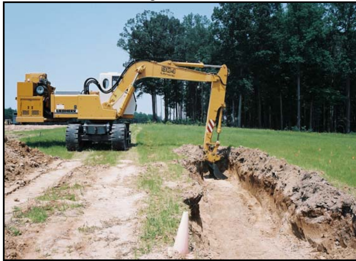
Figure 7. Working Across Trench
